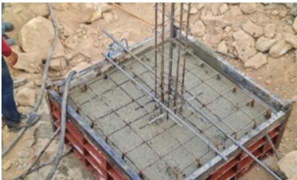
Concrete reinforced with steel bars (rebar)
