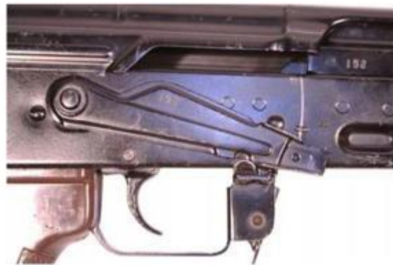
Figure 7. The Selector Lever Placed on SEMI.
